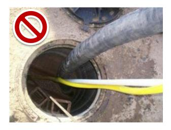
A hose with a severe cover cut, probably produced by sharp edges inside the sewer.
